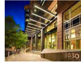
530 COLLINS ST MELBOURNE CBD
